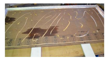
Once Mounting strips, borders and Rosettes are securely in place 'check measure' the space for the centre panel, trim panel, corners etc if necessary.
