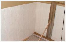
6. Continue in the same fashion with your next panels, running a bead of silicon along the edges of the panels, overlapping joints as you go along and up the walls. Joins will require a Sealed pop rivet to secure in place, these can then be touched up to match powder coat colour at a later stage.
