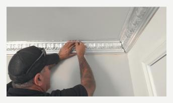
8. Fill the join with paintable No-More Gaps® and smooth this over with a wet paint brush for a clean finish.
