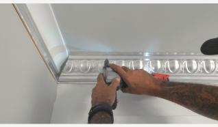
7. Repeat the process for the left-hand cornice. Fine tune until you're happy with the corner join - a gap of around 5mm is fine.
