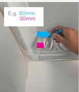
6. Trim with tin snips and fix this cornice to the ceiling using the drill and long shank pop rivets along the edge as required.
