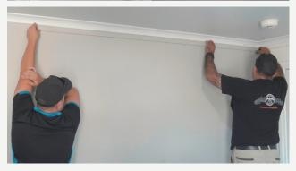
NOTES: If you are going over an existing cornice that is smaller than your new one there is no need to remove the existing cornice, the pressed metal one can be installed straight over the top. Ceiling panels go up after most of our cornices, the exceptions being the Small Plain and the Small Grate cornices.
