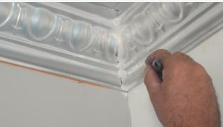
9. **IF INSTALLING WITHOUT EXISTING CORNICE:** The right-hand length of cornice can be installed straight into the corner without the need for trimming. The left-hand length needs to be scribed/trimmed as above to the profile of the right-hand cornice.
