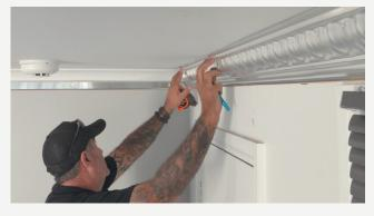
4. The next lengths of cornice overlap the previous ones by around 10-40mm depending on cornice, making sure to pattern match. Overlaps should run away from the eye.
