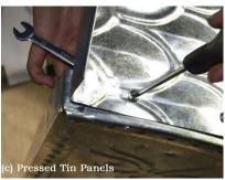
NOTE: Each individual installation varies. Some manual manipulation may be required e.g. tapping along panel edges with the hammer, extra.
