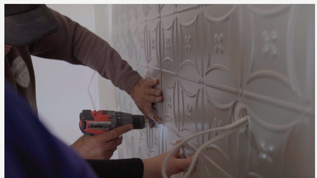
Above example: Pop riveting into place
